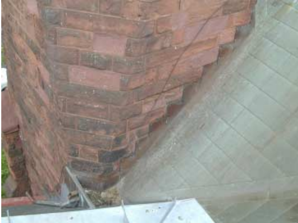
Figure 017: Photo showing drainage collector at southwest corner of west tower
