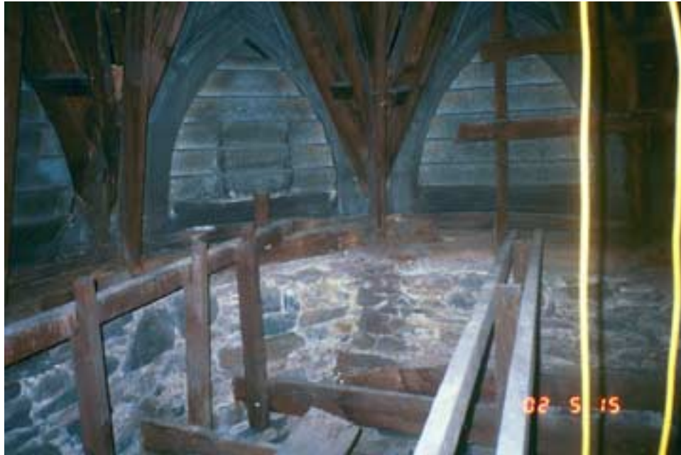
Figure 029: West Tower - Photo showing typical cross section of interior of tower at level of spire
