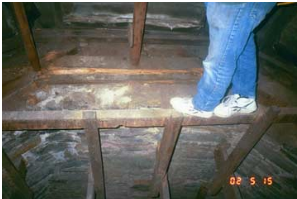
Figure 028: West Tower - Photo showing generous stone ledger suitable for repairing structural damage
