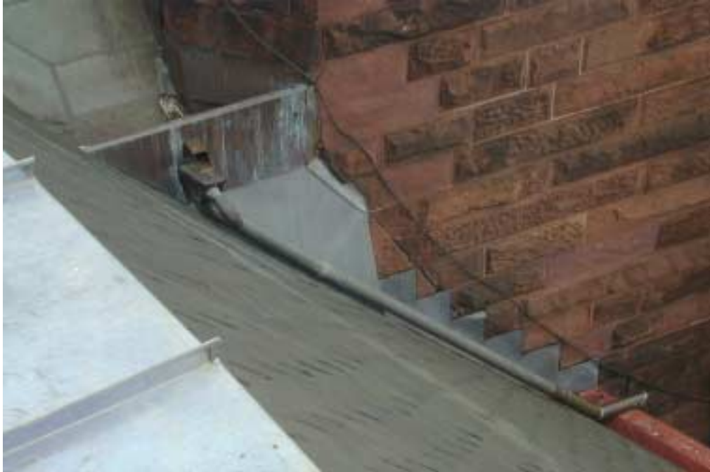
Figure 015: Photo showing Flashing and downspout along face of southeast side of east tower
